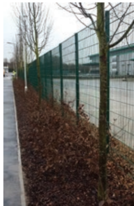
WELD MESH FENCING TO SERVICE YARDS
