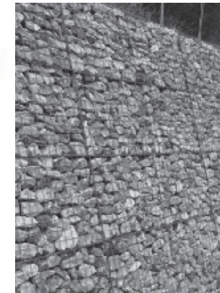
GABION WALL RETAINING IN PUBLIC REALM
