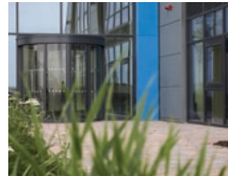
PAVING TO ROUTES TO AID WAYFINDING AND IDENTIFY ENTRANCES
