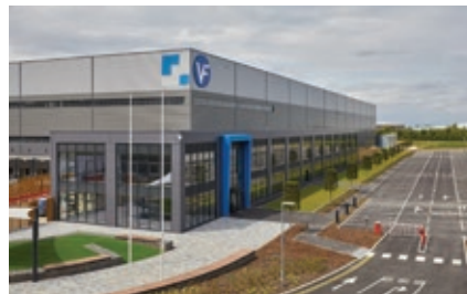
CAR PARK LOCATED ALONG OFFICE ELEVATION
